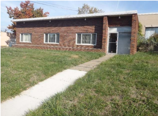
Front of Unimatic Site Building
