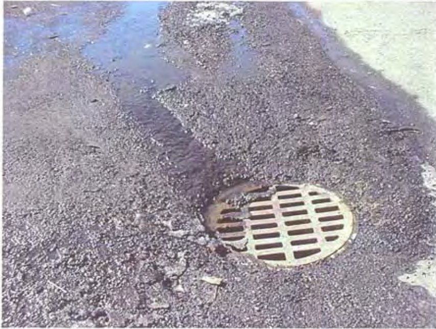
Photograph 13: Storm drain located on the driveway shared between Standard Chlorine and the former Diamond Shamrock site
