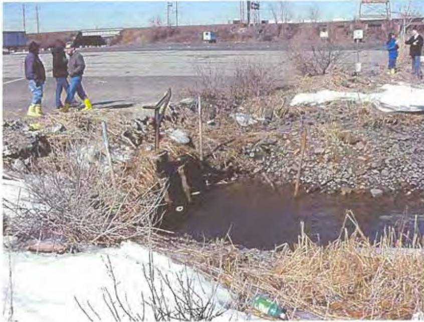
Photograph 11: The north outfall adjacent to the former Diamond Shamrock site
