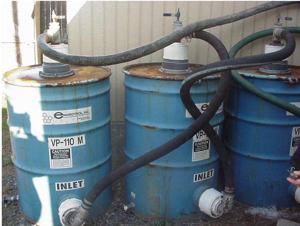
Photograph 5: Vapor-phase carbon treatment drums for the sub-slab vapor recovery system located on The City Grill property.
