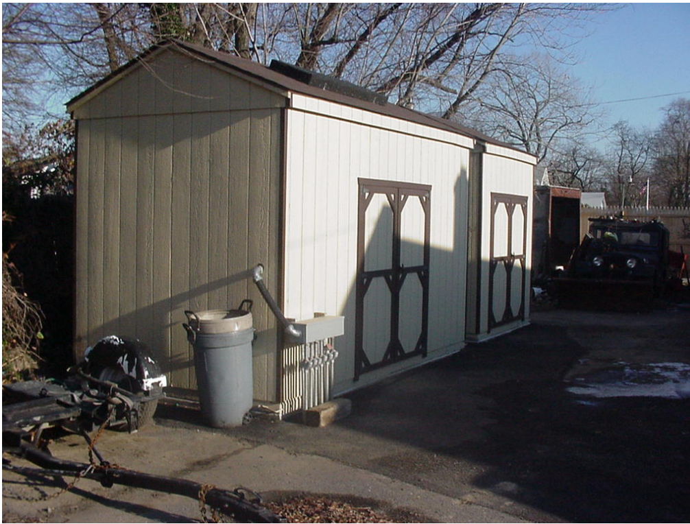
Photograph 3: Groundwater treatment system on the Sal's Auto Repair site.
