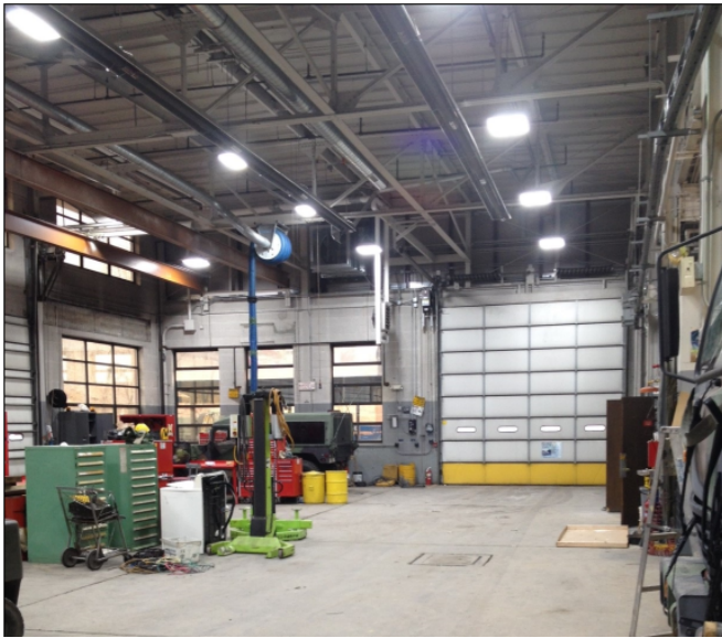
New LED fixtures light up a vehicle maintenance bay at West Orange CSMS.
