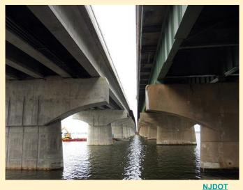
When the Manahawkin Bay Bridge span was replaced, a concrete beam bridge (left) replaced the steel girder bridge (right).
